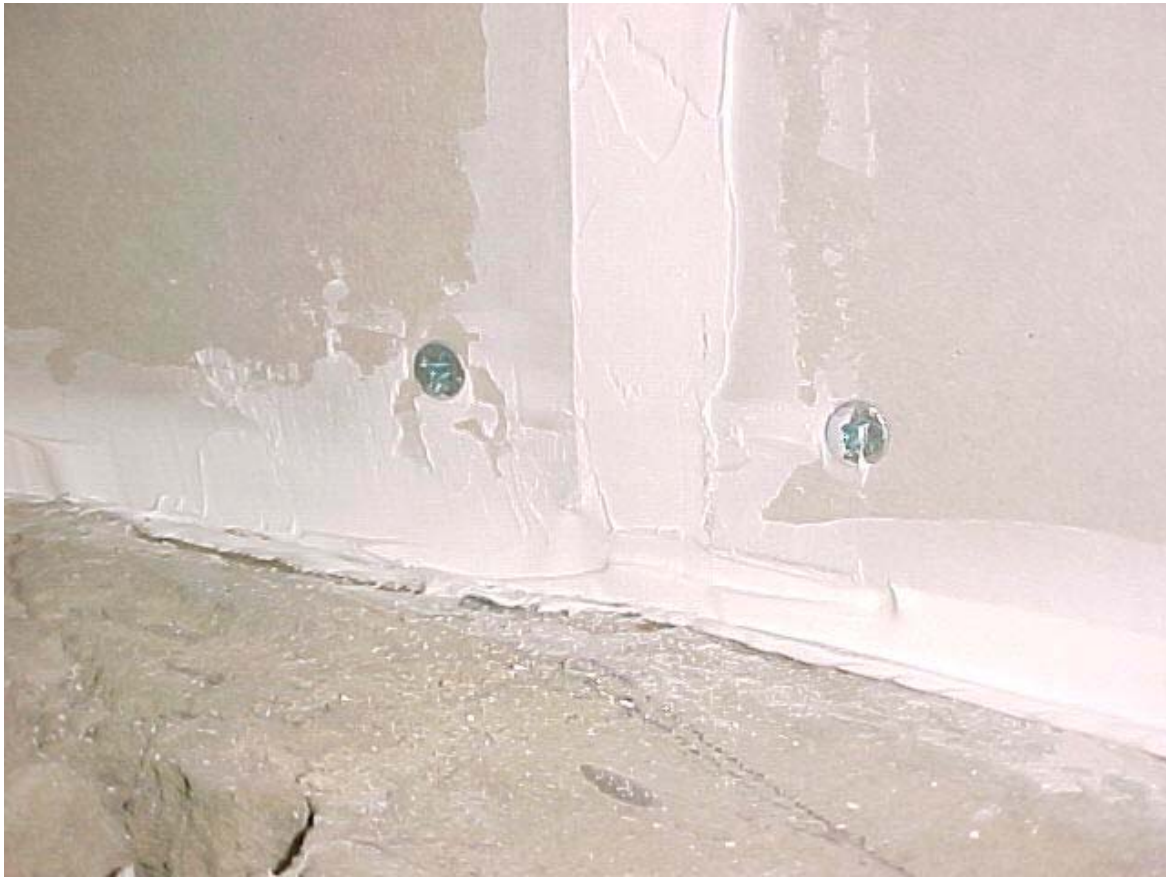
Photograph 4: Fully Sealed Partition Close-Up
